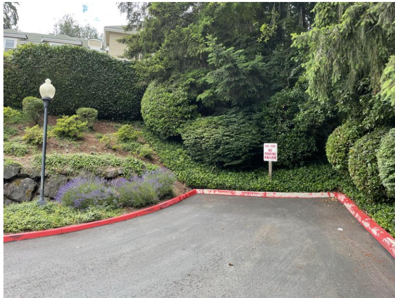
Photograph 1. View of the fire lane and the location of the proposed concrete generator pad. Looking west.
